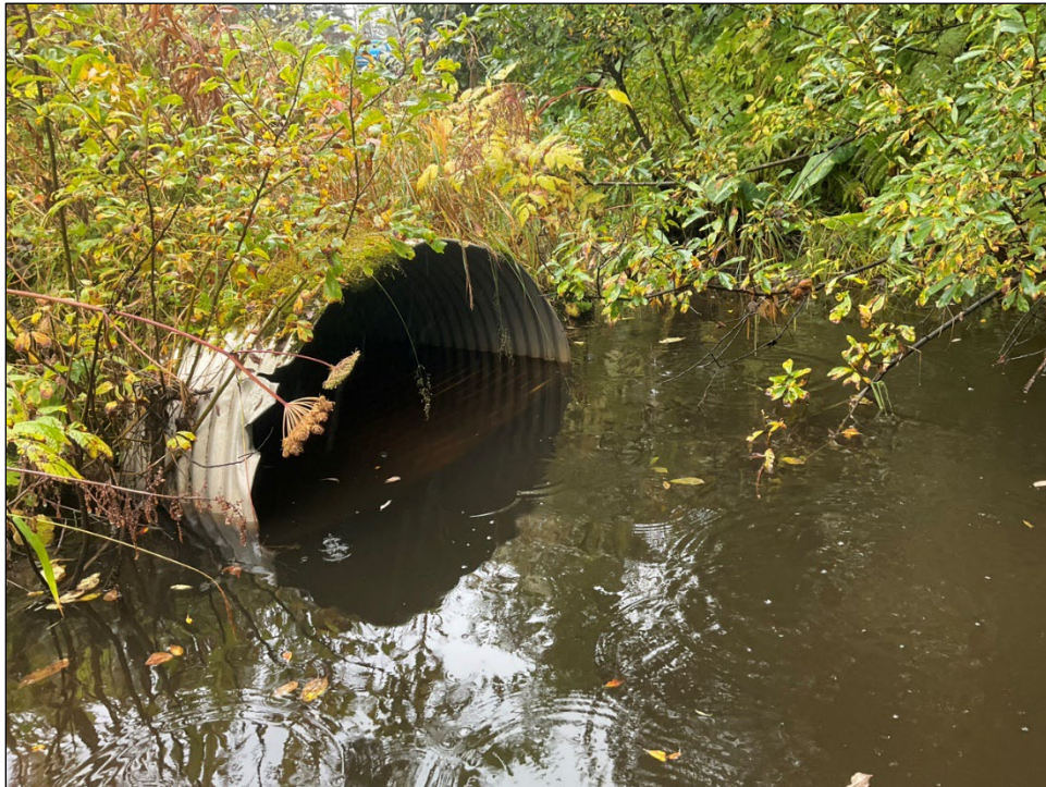
Figure 3.—5ft culvert at waypoint 1248.
